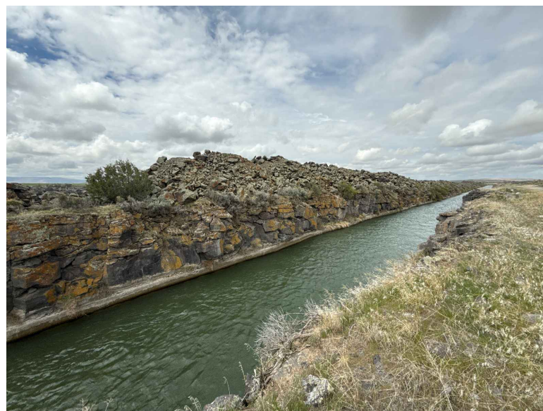
3 REPRESENTATIVE PHOTO OF EXISTING ROCK STOCKPILE ON SOUTH BANK. TAKEN AT APPROXIMATE STATION 45+00
