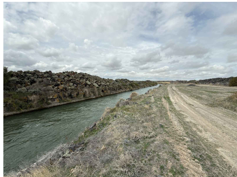
2 REPRESENTATIVE PHOTO OF EXISTING ROCK STOCKPILE ON SOUTH BANK. TAKEN AT APPROXIMATE STATION 61+00
