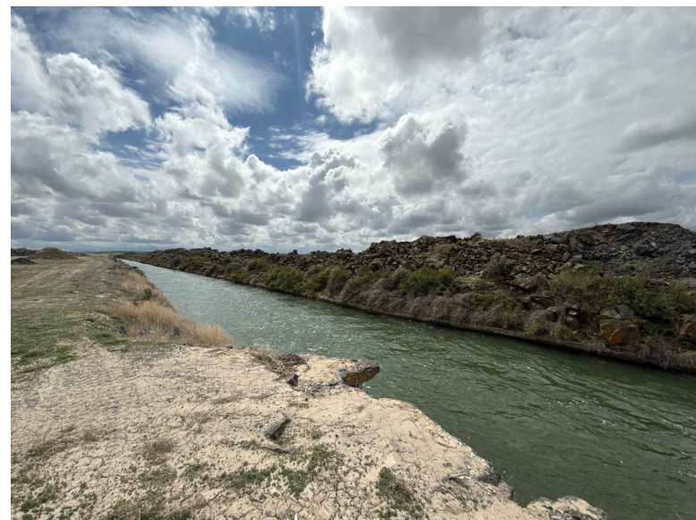
1 REPRESENTATIVE PHOTO OF EXISTING ROCK STOCKPILE ON SOUTH BANK. TAKEN AT APPROXIMATE STATION 70+00
